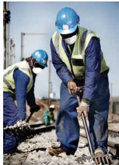
Construction under way at the Port of Ngqura
