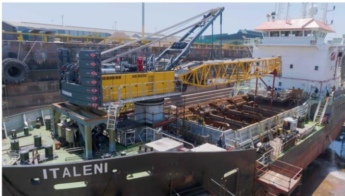
Grab Hopper Dredger – Italeni after upgrade of Marine Excavator
